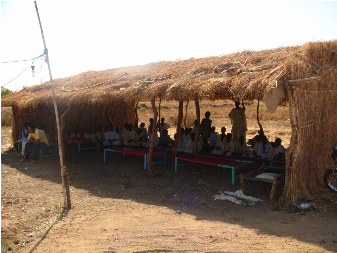
A grass thatched rakuba serving as the classroom, reception and dining hall.
