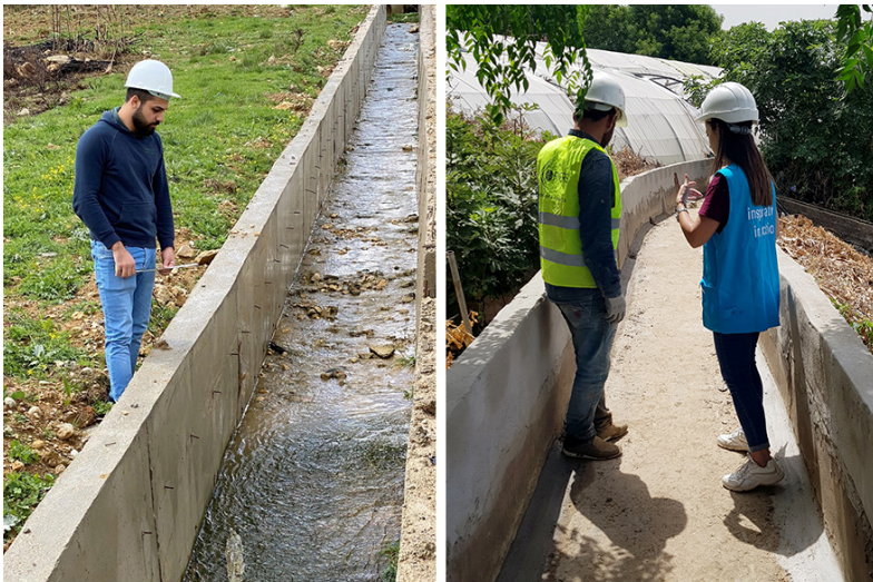
UN Youth Volunteers Nizar Mortada (left) and Raymonda Chamoun (right), examining works on rehabilitation of irrigation systems in Bekaa and Amchit, respectively. © UNDP Lebanon, 2019
