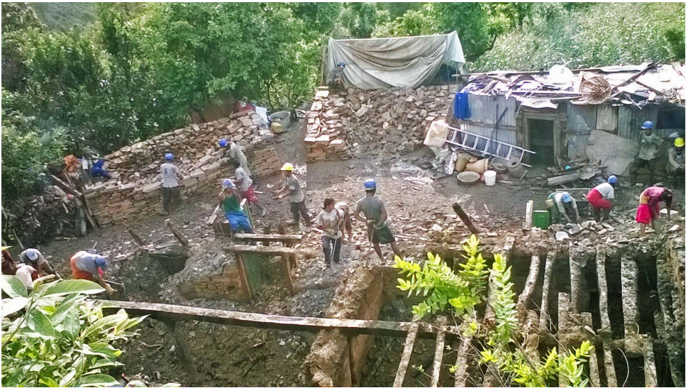
Volunteers working in the UNDP Demolition and Debris Management Project in Nepal in 2015.
