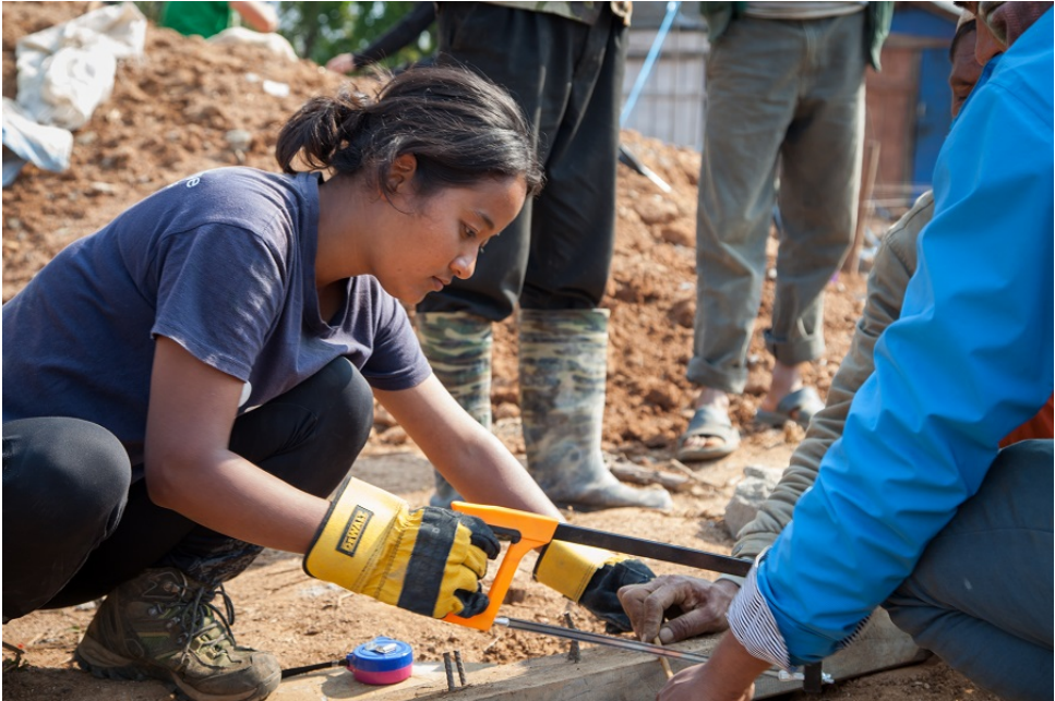
Preity worked with international volunteers on a house-building project (2015).
